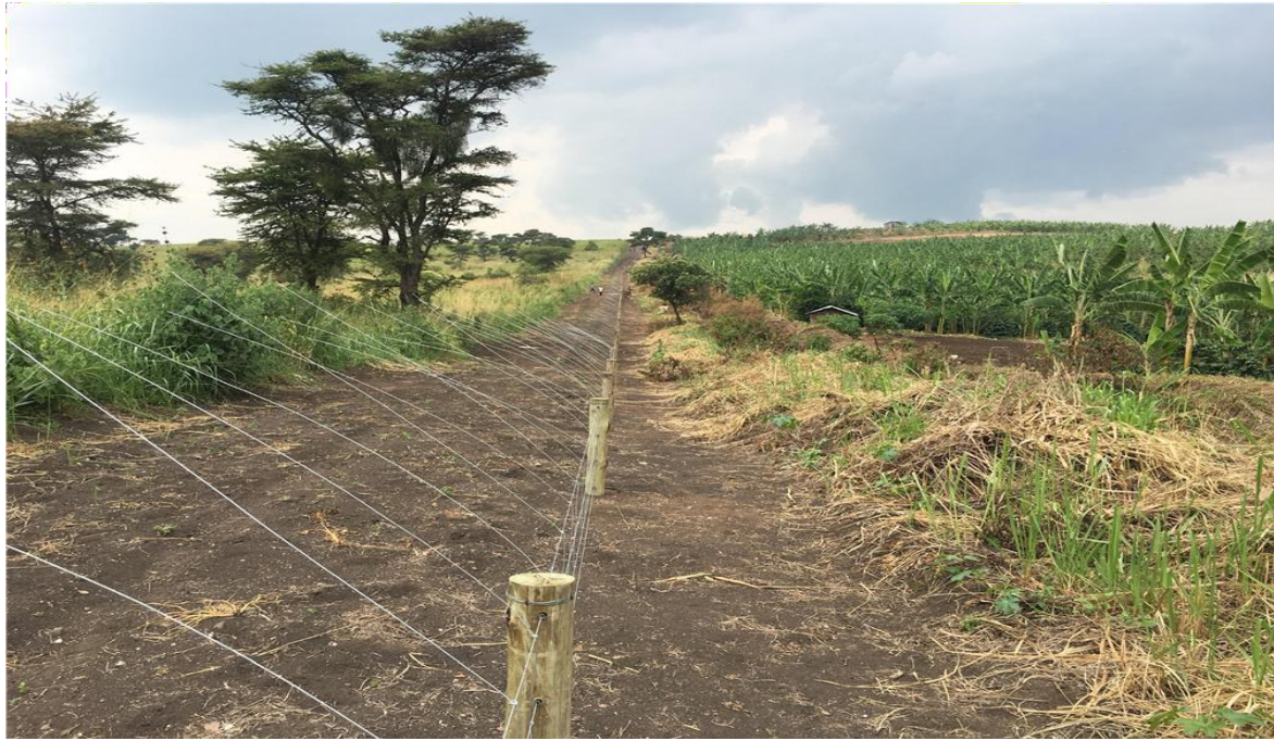
Figure 23: Electric fence in Kyenzaza -Kagarama (QENP)
