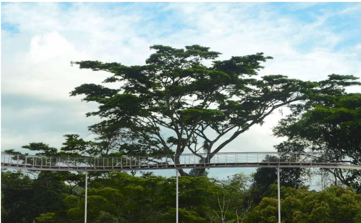
Figure 2-12: Canopy walk supported at 12m intervals
