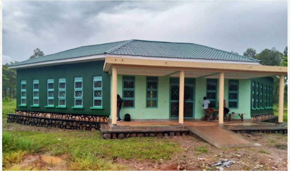
Nearing completion: Office building at Mbale satellite zoo
